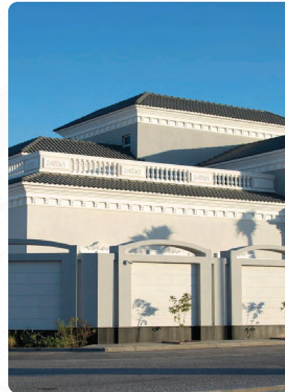
Restoration of residential villas
